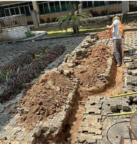
Unified Upgrading of Water Pipes in the Owada Park
