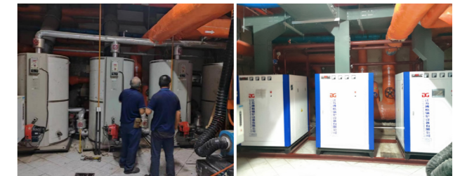
Before and after boiler retrofits
