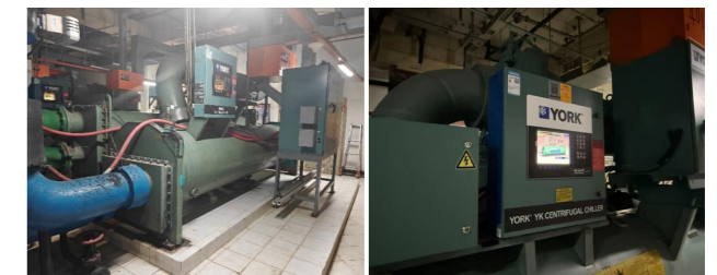
Before and after chiller unit retrofits
