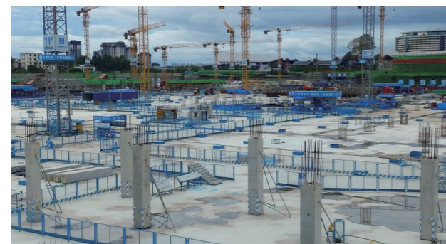
^ The Sanya International Duty-Free Shopping Complex Phase 3 Project utilises a "prefabricated beams and columns with composite slabs" approach.
