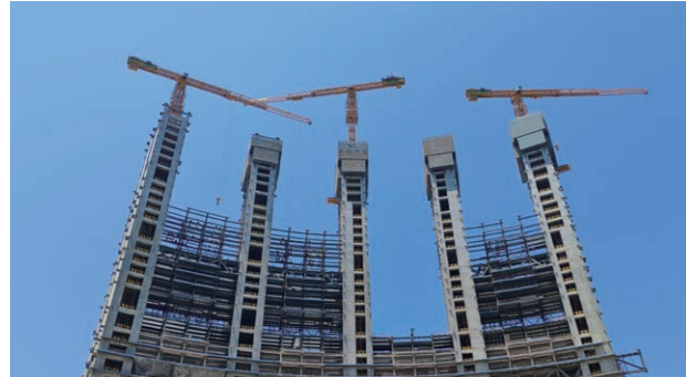
^ The Sanya International Duty-Free Shopping Complex Phase 1 Hotel Project employs a "steel truss with reinforced concrete slabs" method.
