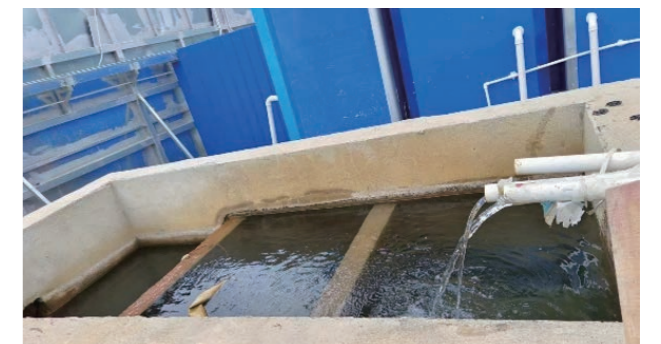
^ Implementation of rainwater collection devices on construction sites for recycling rainwater and construction drainage
