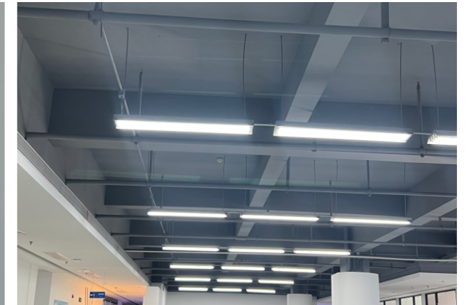
Replacement with energy-efficient LED lighting
