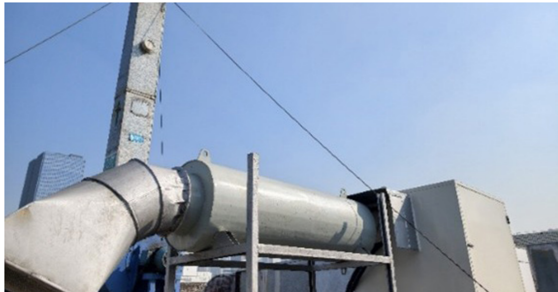
Precise Position Hazard Prevention and Equipment Upgrade Noise Reduction Renovation
