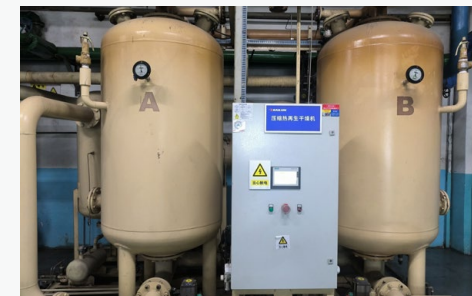
Compressed Air System Retrofitting at Shenyang Factory
