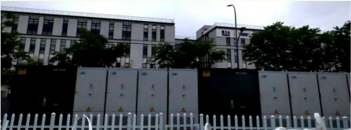
Photo of New Project Plant
