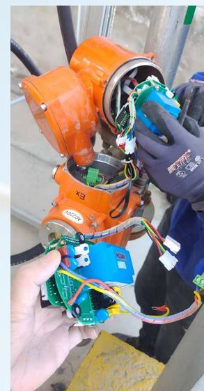
Repair of the Explosion-Proof Electric Adjustment Actuator
