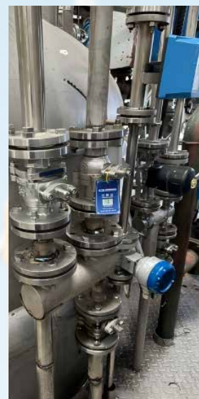
Polishing, Cutting, and Reusing Stainless Steel Pipes
